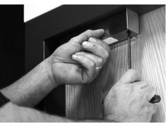
Figure 17. Installing the Magnalock
