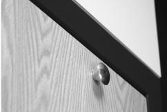
Figure 15. Installing the Sex Bolt
