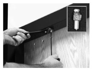
Figure 9. Installing the Blind Nuts
