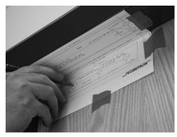
Figure 5. Marking Drill Hole Locations
