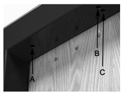
Figure 7. Lock Body Drill Holes
