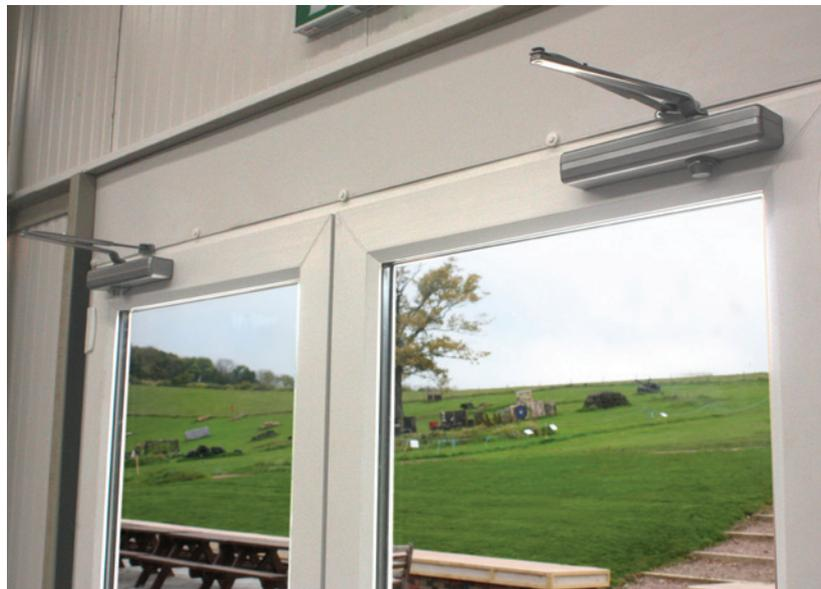
120 minutes or (steel) 60 minutes. The extra power and robustness of the LCN closer means the wind affected doors now close properly and securely eliminating the previous problems and ensuring Hillside Brewery maintain their green credentials.
